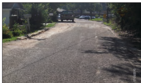
East Alabama Street (Before)
