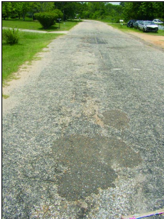
Pictured above is Friar Road before the paving project.
