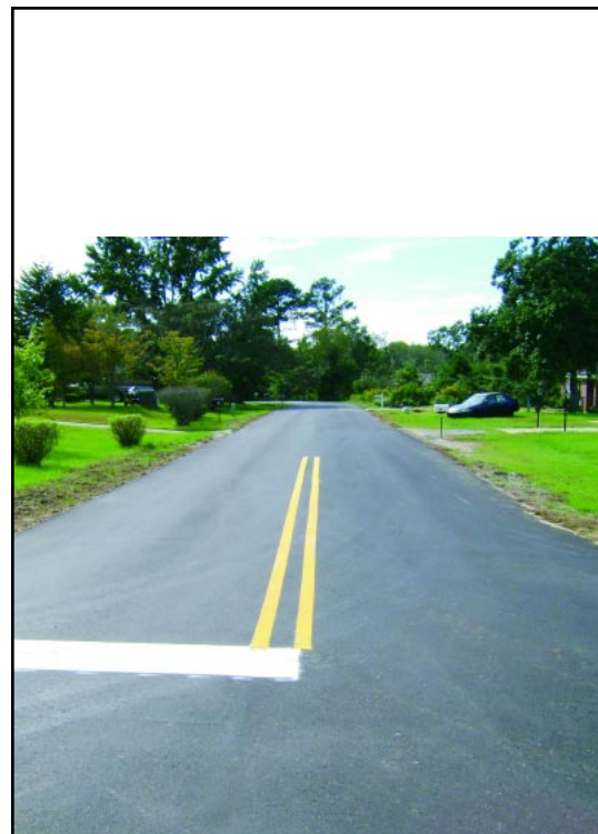
Pictured above is Friar Road after the completion of the paving project.
